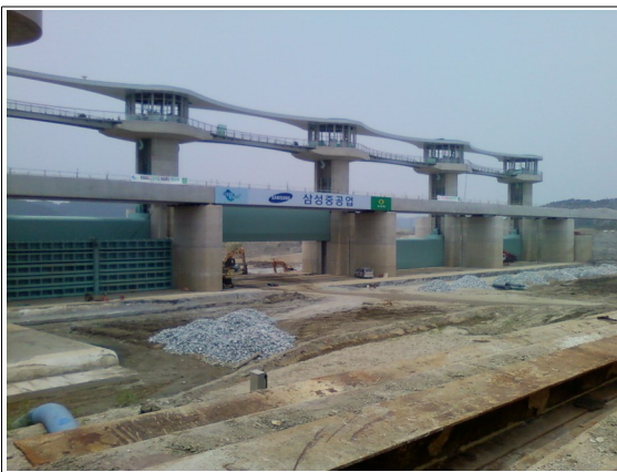
Pic 1: Floodgates under construction
